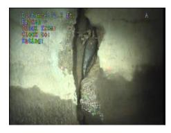
From/To Code Modifier/Severity Distance Dir. Length Rating Comments 72.9 ft. 7/ D Crack Crack D 5 /
