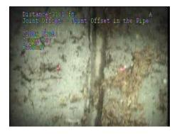
Distance Dir. Length From/To Code Modifier/Severity Rating Comments 9 / 31.1 ft. U Crack 39.2 ft. U Joint 1 39.2 ft. U 11 / Chip Broken
